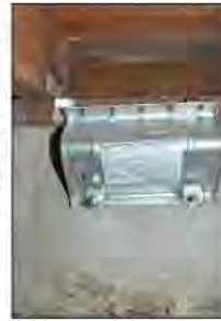
Foundation hardware connecting mudsill to foundation wall.
