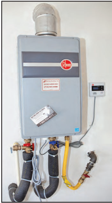
The Lennar home design comes with low-emissive, or 'low-E,' glass windows, seen here, which stop heat from entering the home and reduces the use of air conditioning. At left, Lennar offers preinstalled tankless water heaters, which cut down on energy consumption by only heating water when necessary, in addition to other features. (Photograph by the Business Journal's Thomas McConville)
