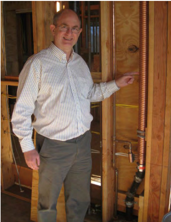
Hot water expert Gary Klein shows the upstairs Power Pipe Drain Water Heat Recovery Unit.
